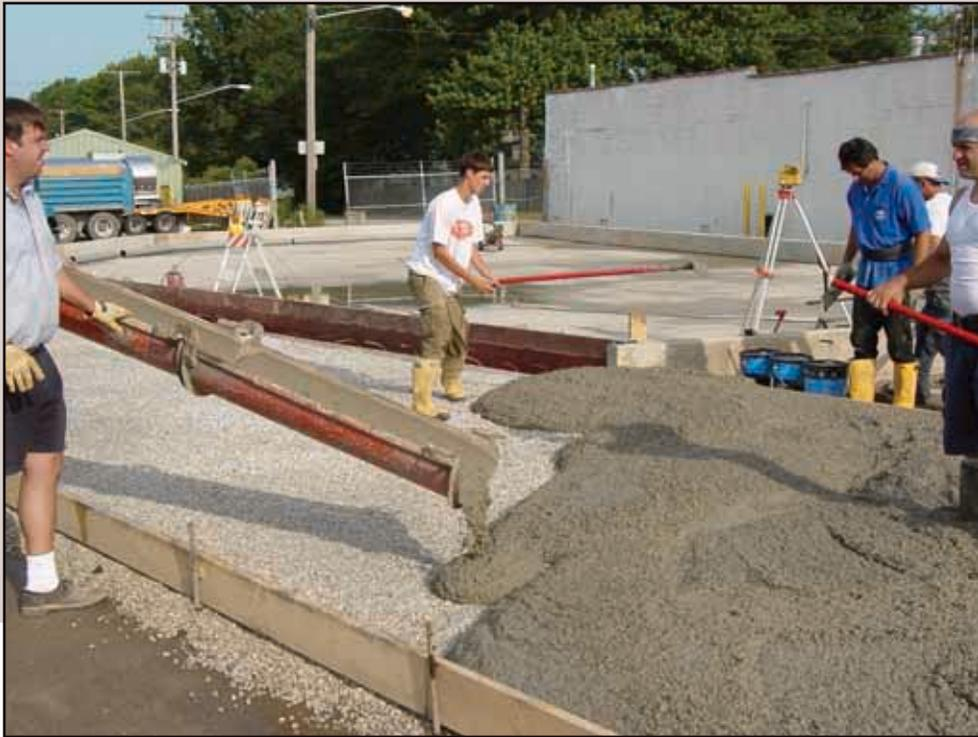
The reinforced concrete being poured in this photo contains macro-synthetic material capable of producing similar toughness to steel fibres and light-gauge rebar. As an increasing number of manufacturers and distributors are marketing these products, the various technical organizations are trying to develop approvals, practices and guide specifications.
