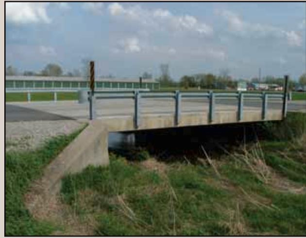
*A concrete bridge repair project in Howard, Wis., used synthetic fibres to gain resistance to repeated freeze-thaw cycling.*
