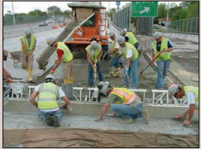
*Advancements in extrusion properties and polymer production have yielded synthetic materials providing similar performance to steel fibres. They can be added at higher reinforcing levels to offer enhanced toughness. The above photos show the placing and finishing of this fibre-reinforced concrete (FRC).*
