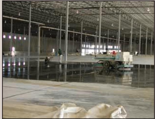
On the left, a close-up illustrates the smooth final finish of a macro-synthetic fibre-reinforced concrete slab. The photo on the right depicts the application of surface sealer on a newly placed slab.
