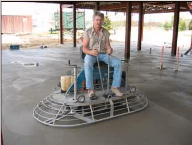
Power troweling a freshly placed macro-synthetic fibre-reinforced slab at Bishop's University in Lennoxville, Que.
